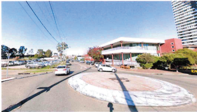
4 View Along Prince Street looking South
